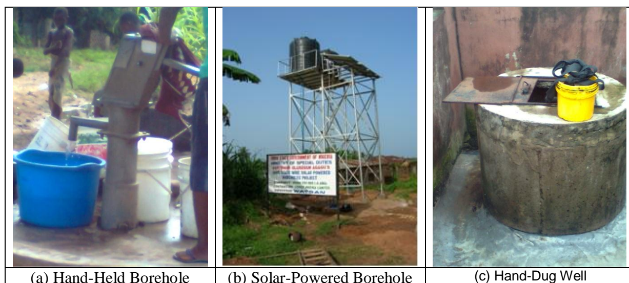
Figure 3. Example of (a) Hand Held Borehole, (b) Solar Powered Borehole and (c) Hand-dug well in the study area.
