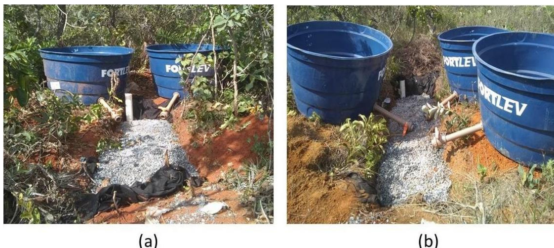
Figure 2. Infiltration Trench in (a) Red Latosol (TR4) and in (b) Red-Yellow Latosol (TR5).
