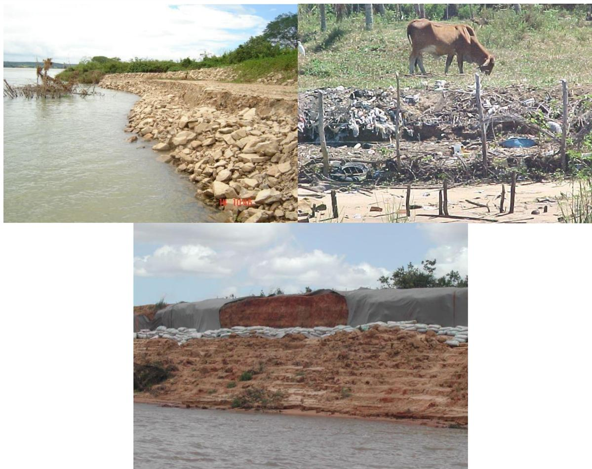
**Figure 5.** Riprap and other erosion-control methods used by the riverine population.
