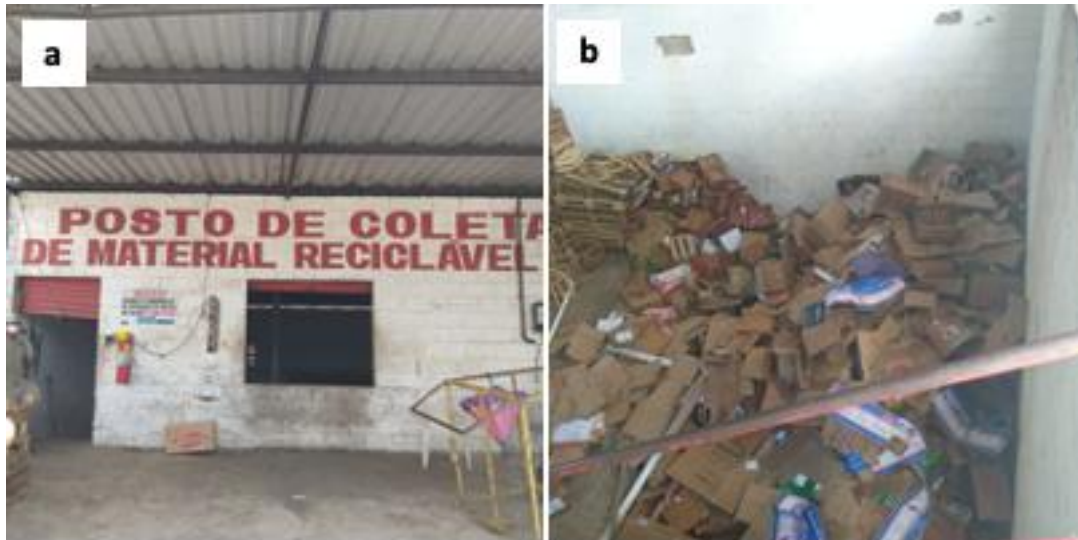
Figure 2. Collection shed for recyclable material at CEASA-MA. External (a) and internal (b) views. Photo by author.
