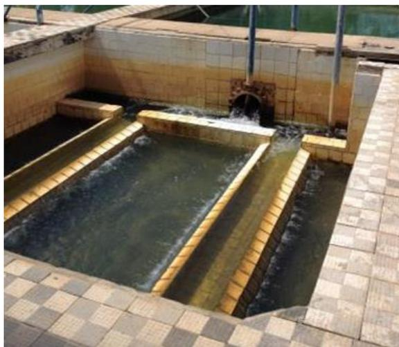
**Figure 1.** Image of one of the filters during the backwash process.
